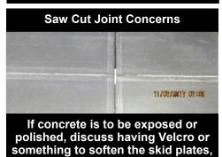
These scratches will NOT go away with polishing the concrete.
